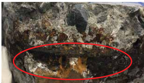
Fig 7. Inside Surface of Concrete Block with Black Bar after Breaking
